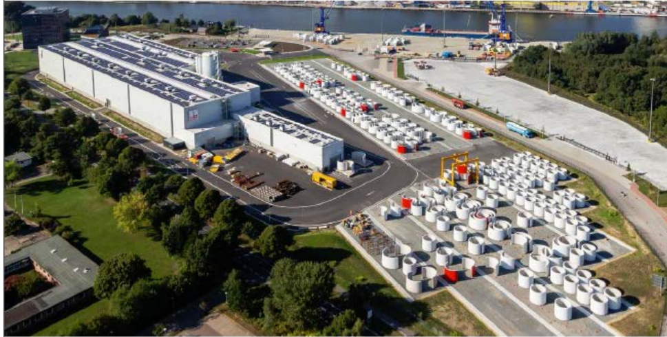
Figure 1.22. Storage of precast concrete components at production facility (Max Bogl, 2016)
