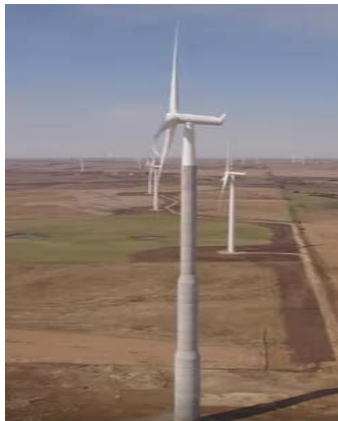
Figure 1.27. MidAmerican hybrid tower (MidAmerican Energy, 2016)
