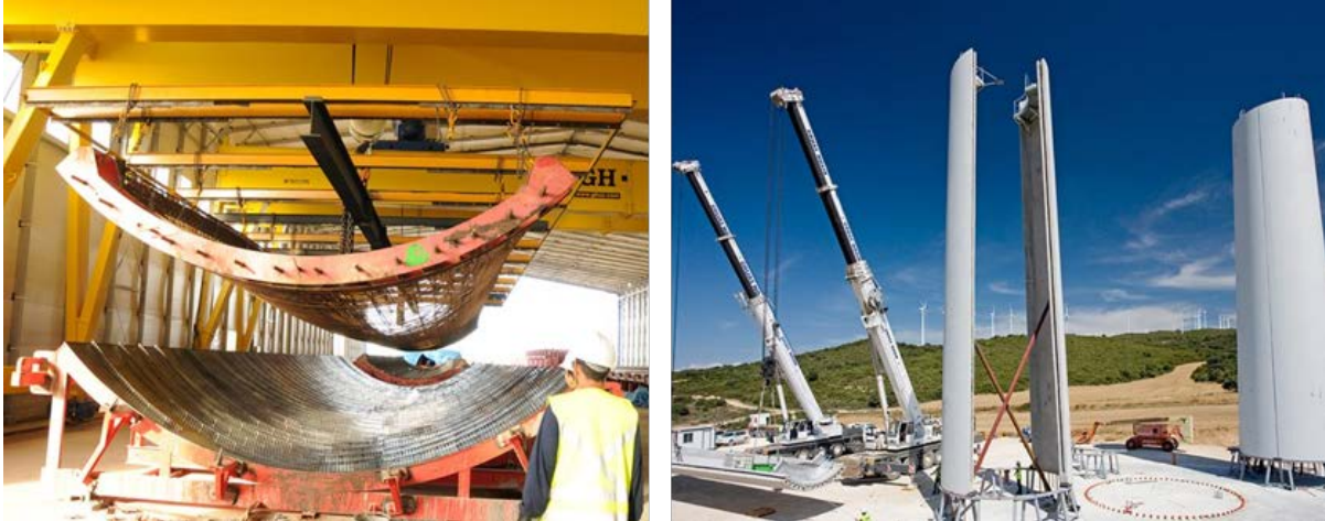
Figure 1.11. Acciona Curved shell formwork (left); shell assembly (right) (Acciona WindPower, 2016)
