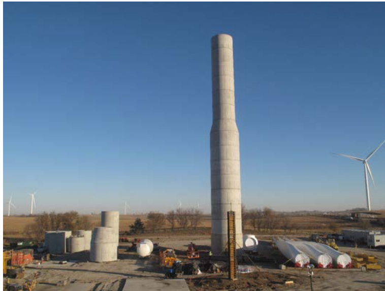
Figure 1.29. Stacked concrete tower sections (MidAmerican Energy, 2016)
