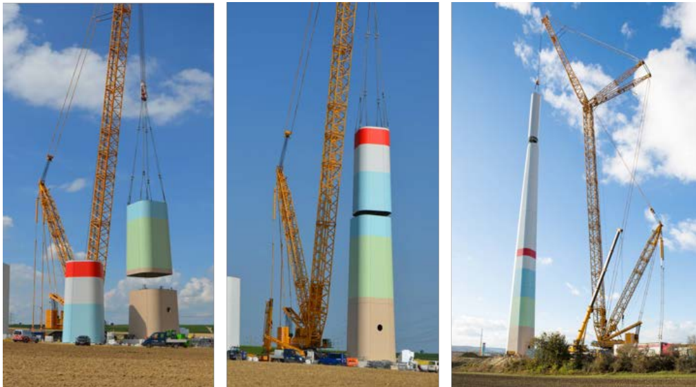
Figure 1.20. Stacking of ATS square concrete base sections (Advanced Tower Systems, 2016)
