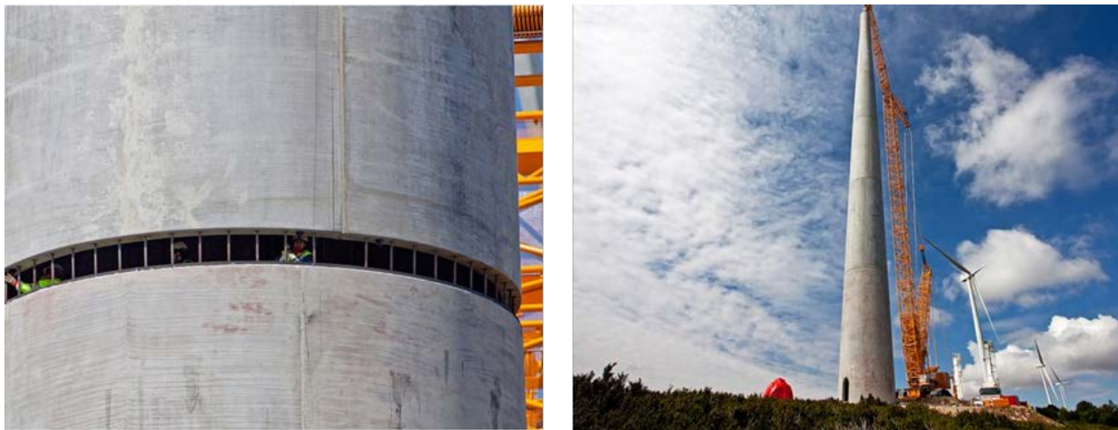
Figure 1.12. Stacking of Acciona concrete tower sections (Acciona WindPower, 2016)
