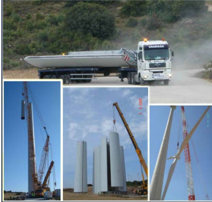
Figure 1.13. Inneo Torres tower transportation and erection (Inneo Torres, 2008)
