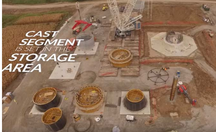
Figure 1.28. Formwork and onsite casting (MidAmerican Energy, 2016)
