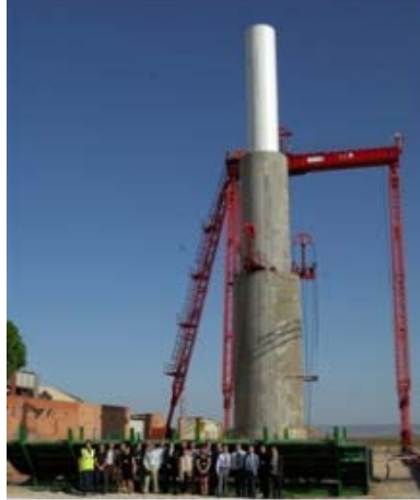
Figure 1.26. Prototype of self-lift Esteyco tower (Esteyco Energia, 2014)
